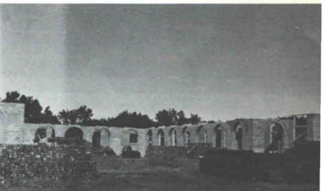
fig. 4 east wing and central portion
