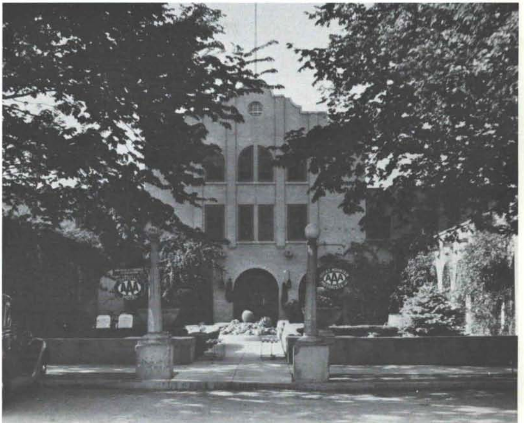
fig. 14 (Fully completed hotel)
