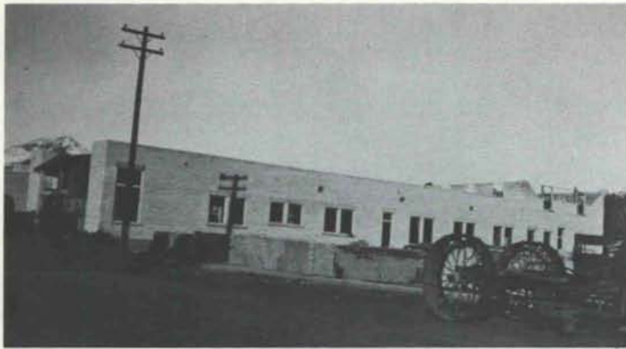
fig. 5 east wing with roof and beginning the second story in the center. Note heavy construction vehicle on the right.
