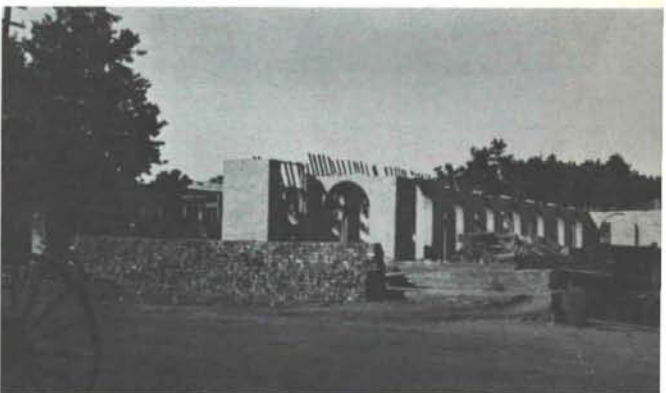
fig. 3 west wing again nearing the top.
